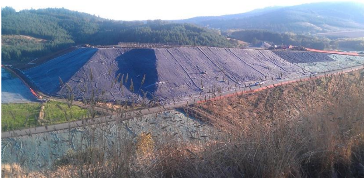
EPDM Geomembrane temporary landfill cover used over a twenty year span, IGS photo contest 2014 (W. Johnson)
