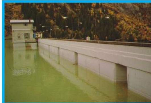
Completed Concrete Dam Lining
