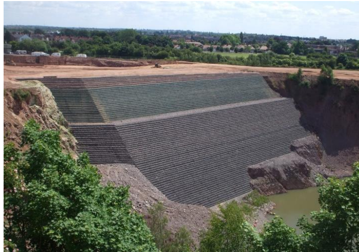
Large reinforced soil just completed, IGS photo contest 2010 (P. Assinder)
