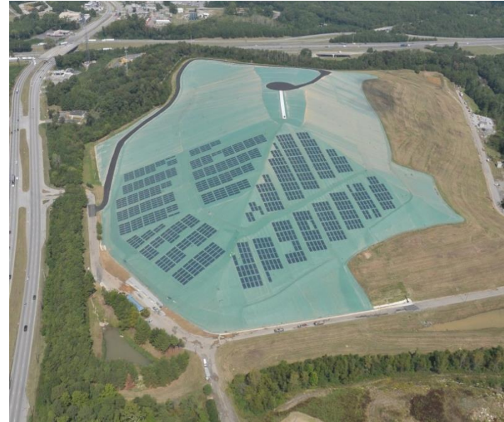
Solar cells installed on an exposed Geomembrane cap at the Hickory Ridge landfill (courtesy Carlisle Energy)
