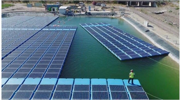
Floating photovoltaic cover (courtesy M. Redón-Santafé)
