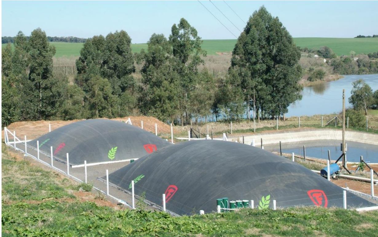
Anaerobic digester lined and capped with EPDM Geomembrane, IGS photo contest 2010 (S. Murray)
