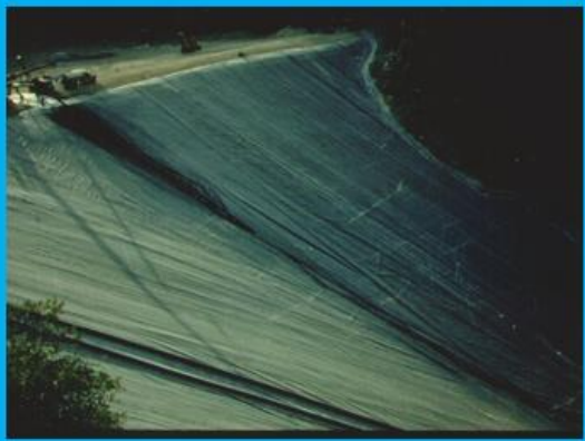
Lined Earth Fill Dam: Before Rip-Rap
