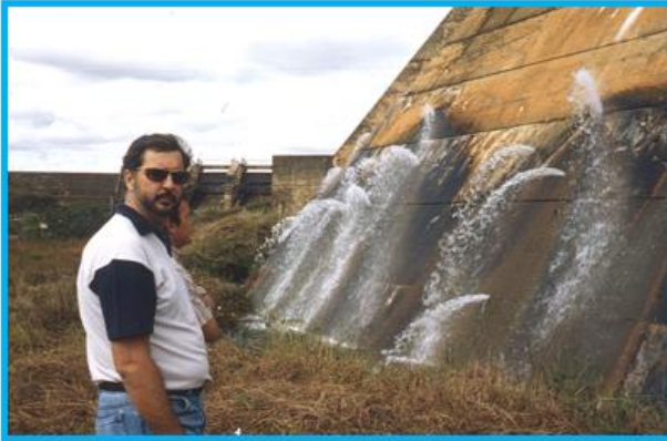
Concrete Dam Leaking!
