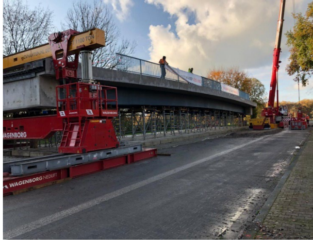
Lift and transport of bridge deck
