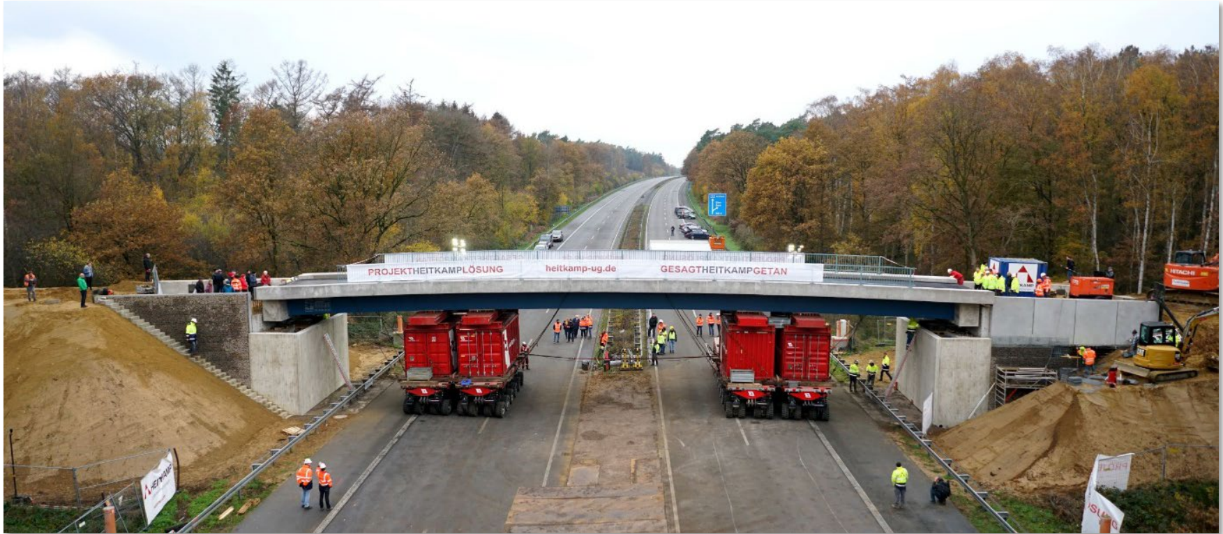
Lift and positioning of bridge deck
