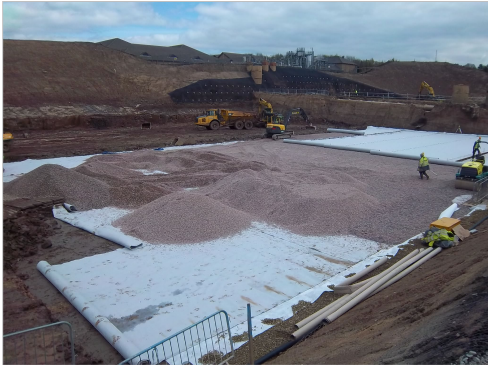
Geosynthetic filter system below a road
